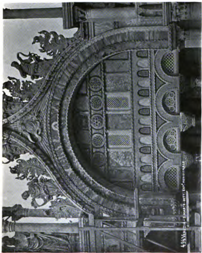
SOUTHERN FACADE OF ST. MARK'S
